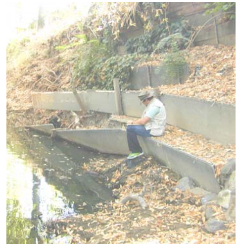
Crib Wall in Alhambra Creek, CA
