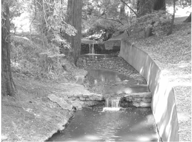
Drop Structures on Strawberry Creek downstream from Sather Gate, UC Berkeley, CA.
